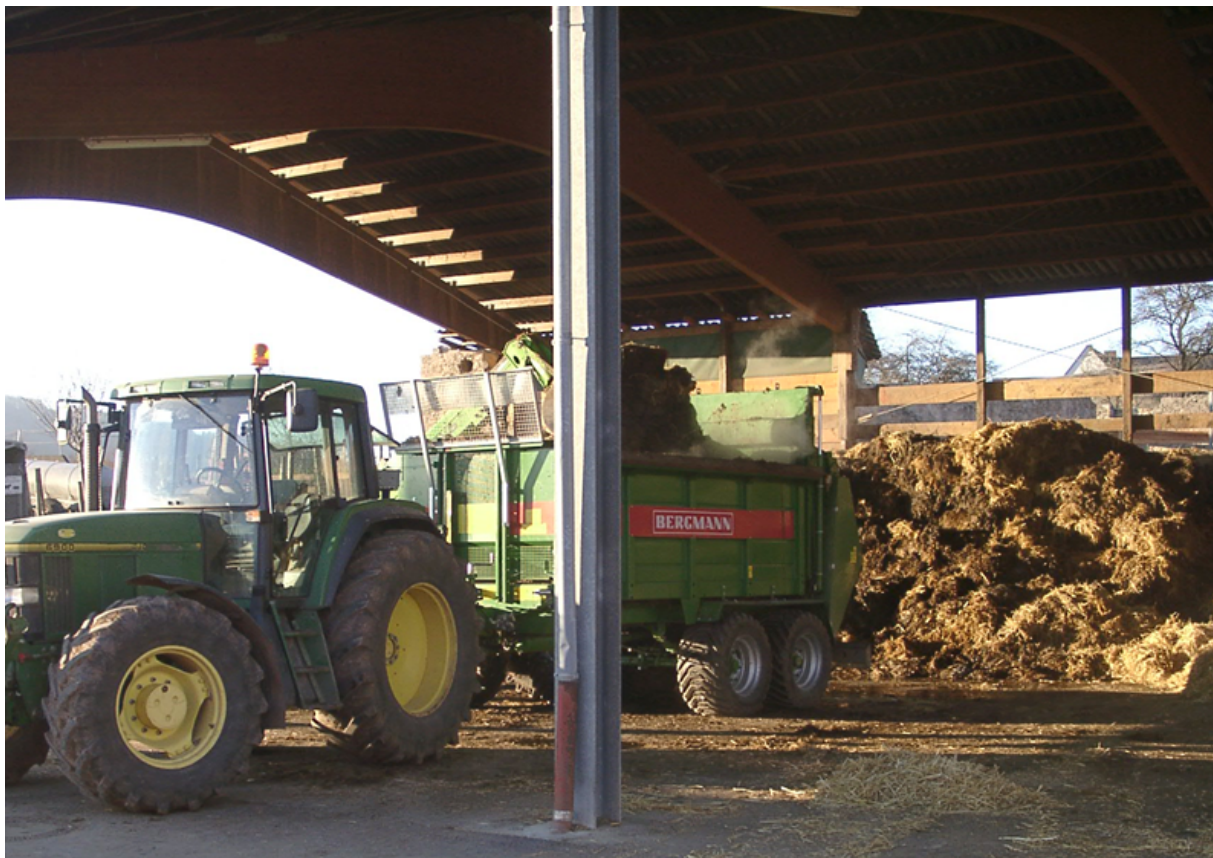
Figure 33: Solid manure storage with permanent roofing
