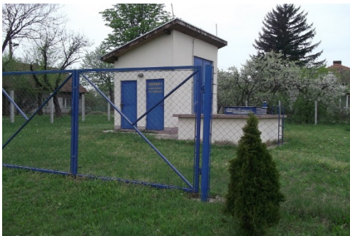
Small water supply in Tornjoš village
