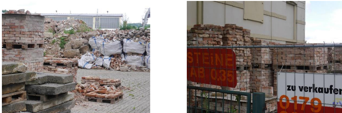
Picture 2: Used bricks before cleaning (background, le.) and piled up for sale after preparation for reuse (ri.)
