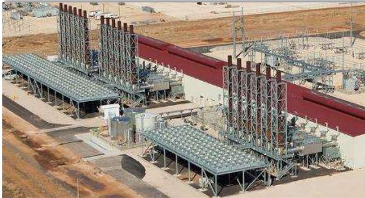
Antelope Power Station, Texas, USA, SCR, 9.4 MW engines
