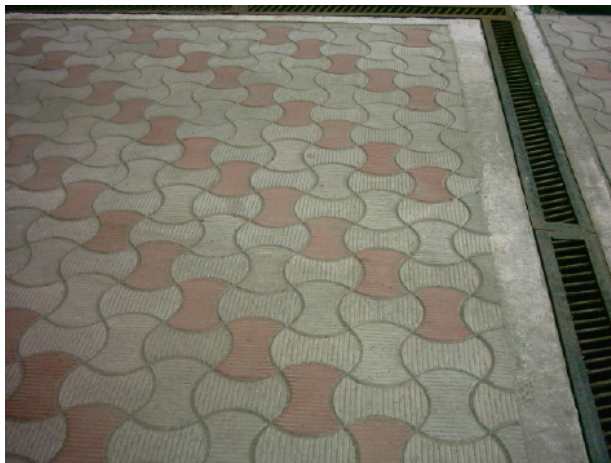
Picture 5: Filling area of the plant's petrol station
