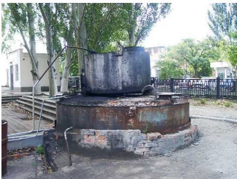
Picture 17: Tank containing a mixture of diesel and waste oil
