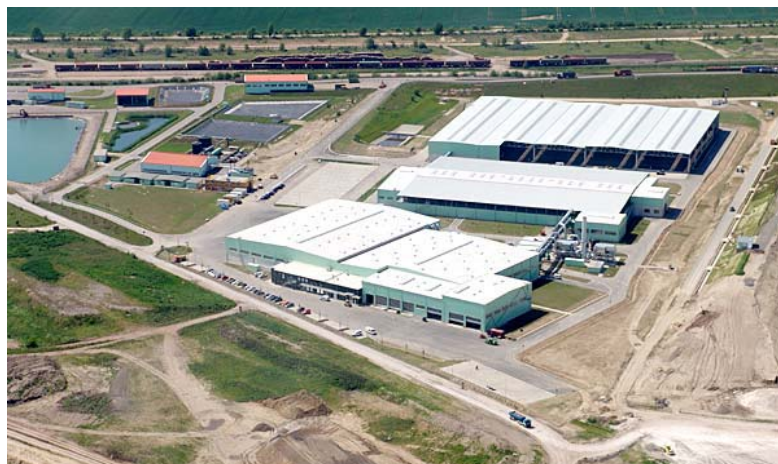
Figure 15 Example of a mechanical-biological treatment plant
