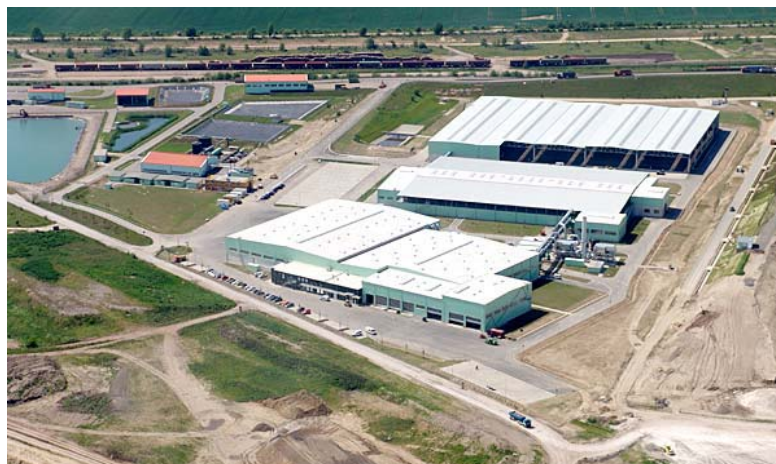
Figure 15 Example of a mechanical-biological treatment plant
