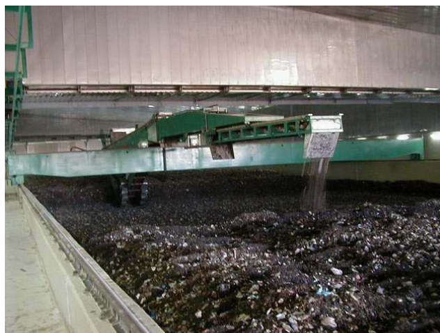
Figure 11 Indoor composting system
