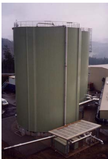
Figure 12 Digestion plant for bio-waste
